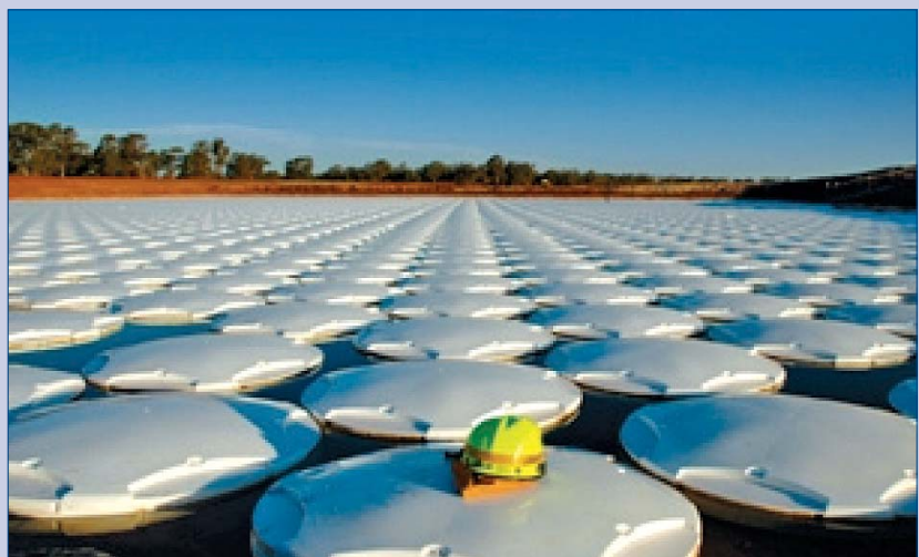
North Parkes, NSW, 2008: Nylex and Rio Tinto joined forces to produce a product that achieved 95% reduction in evaporation losses.
