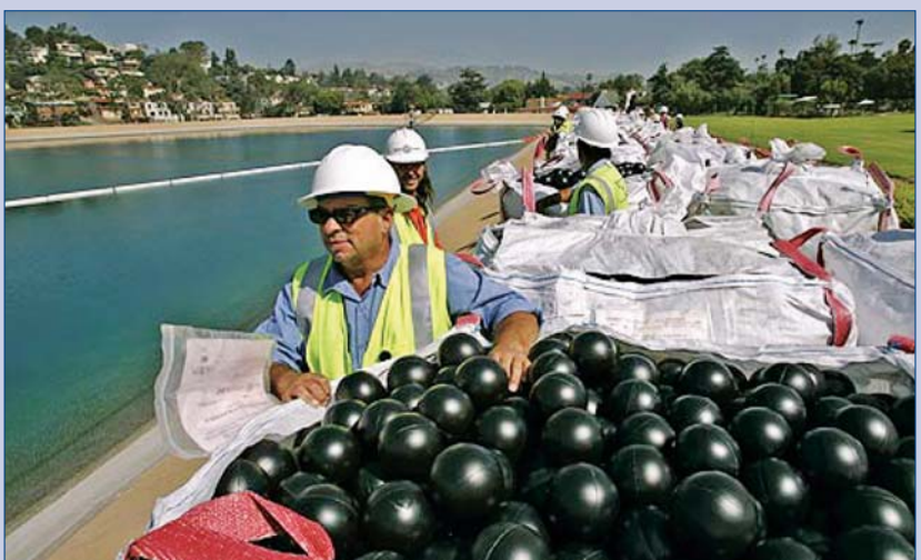
Preparing to spread plastic balls: Ivanhoe Reservoir, Los Angeles, 200 ML, 2007. The water needed to be shaded because sunlight with the bromide and chlorine formed the carcinogen bromate. No reduction in evaporation was targetted.
